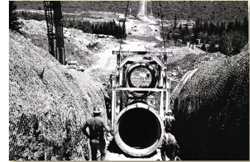
North Fork Siphon on the west slope during the original construction
