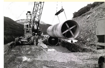
Contractor laying a 40-ft section of the North Fork Pipeline during the original construction
