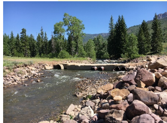
Existing River Crossing Structure
