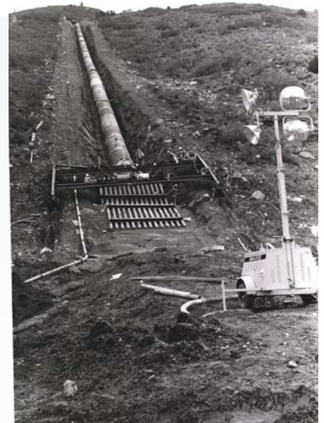
Construction of siphon on east slope.
