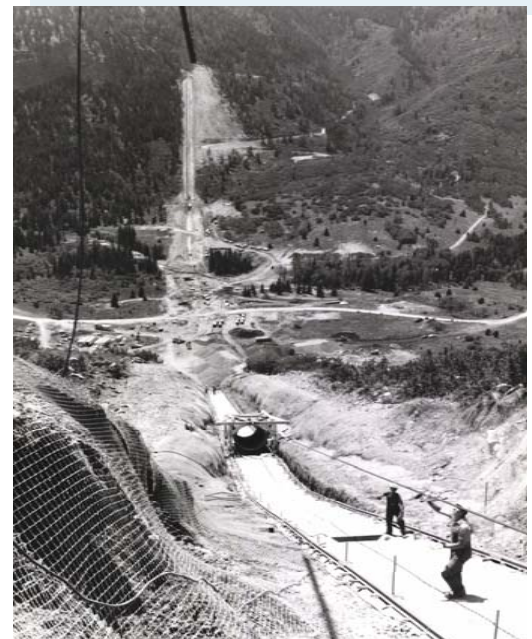
Construction of the North Fork Siphon looking west.
