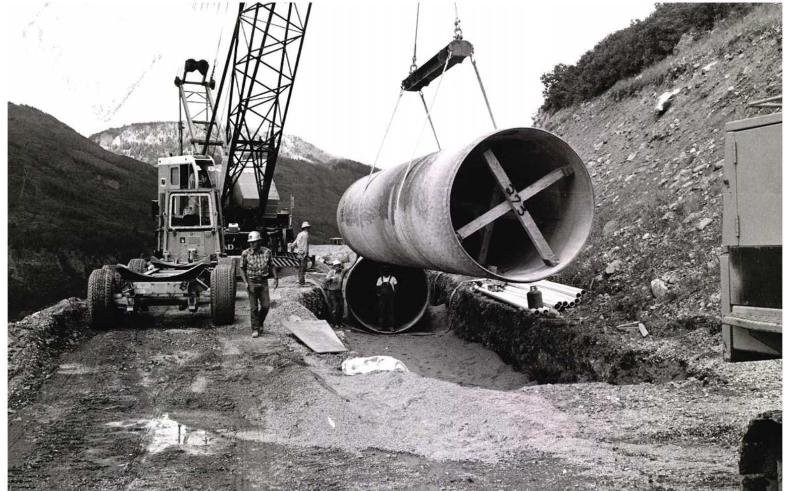
Contractor laying a 40-foot section of the North Fork Pipeline
