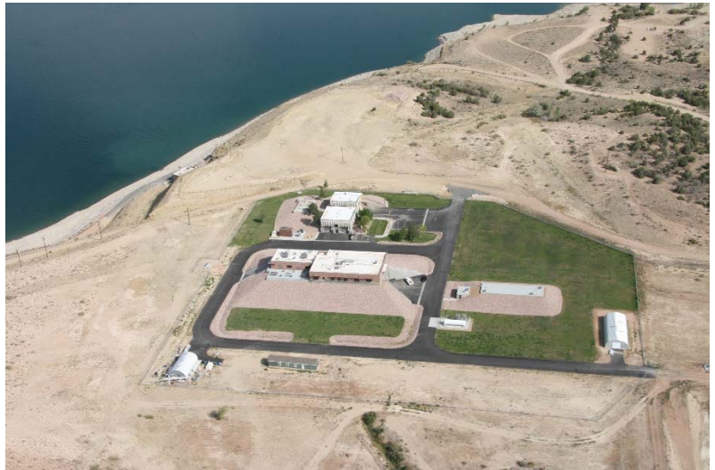
Duchesne Valley Water Treatment Plant
